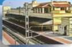
13km - Podanur Railway station
